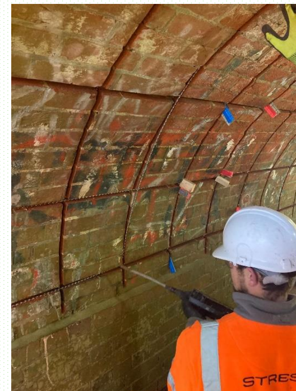
Masonry Arch Repair and Strengthening (MARS) system.
